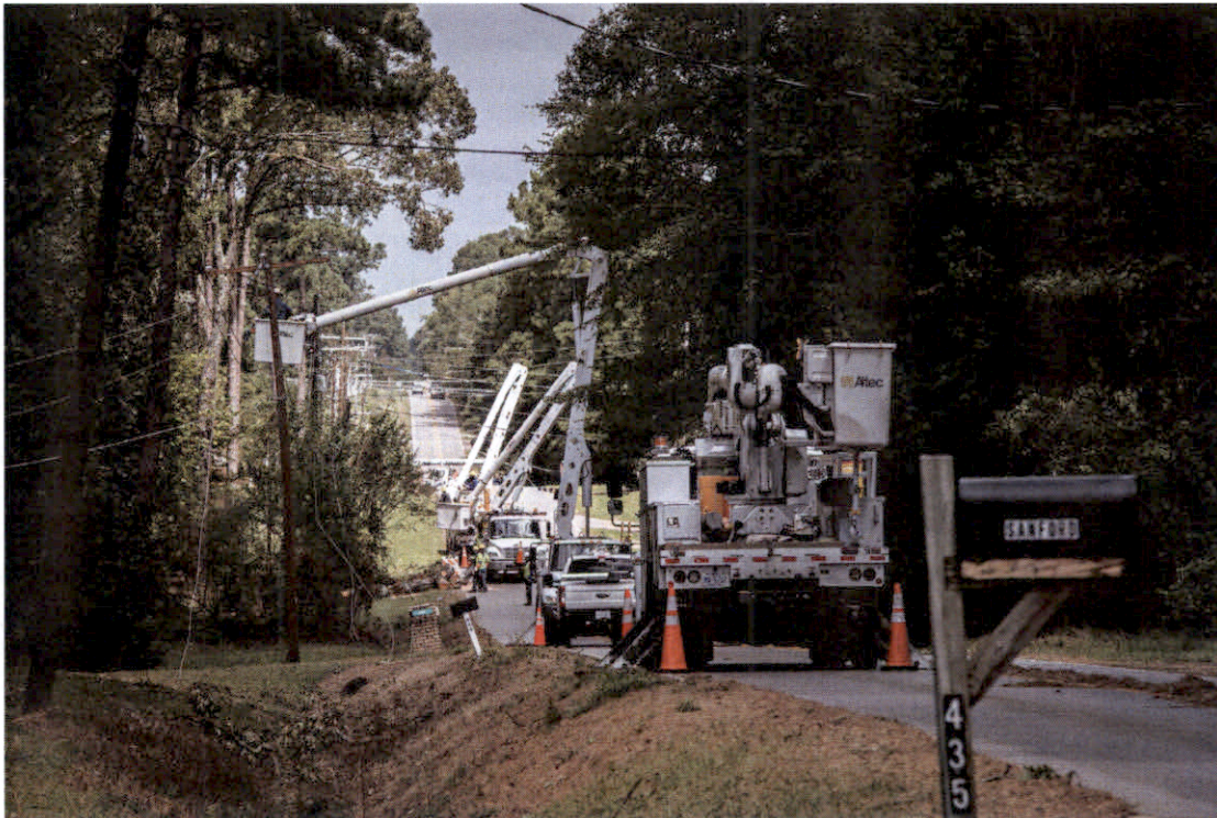
Figure 3 - Crew repairing multiple spans of damaged line and poles
