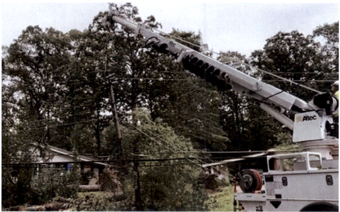
Figure 1 - Crew replacing a broken pole
