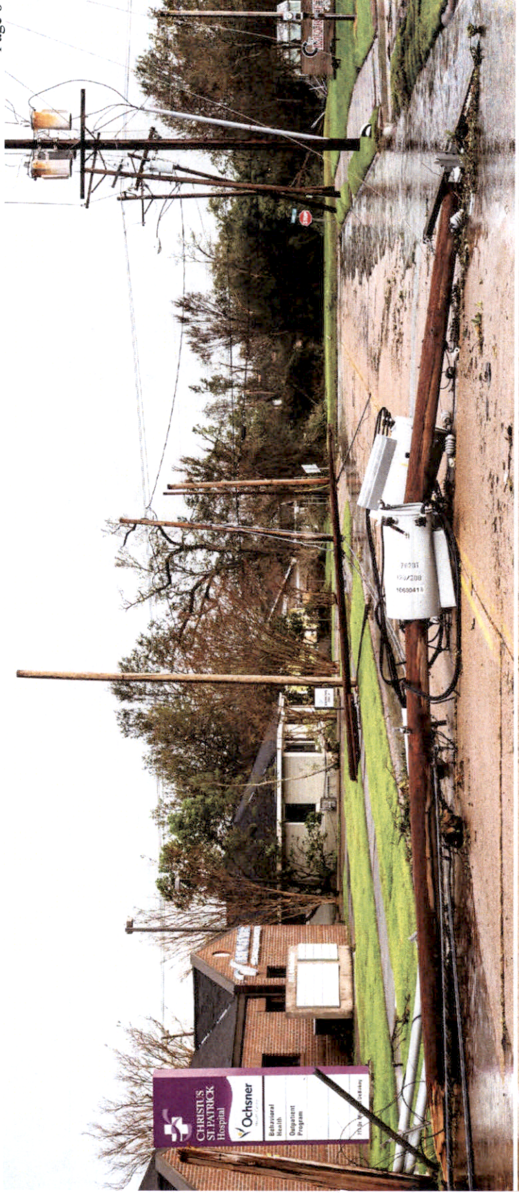
Distribution pole in Lake Charles broken above the groundline
