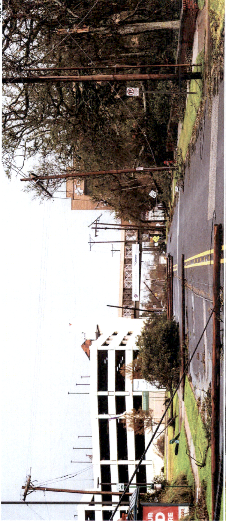
Heavily damaged distribution line, with wood poles broken above groundline
