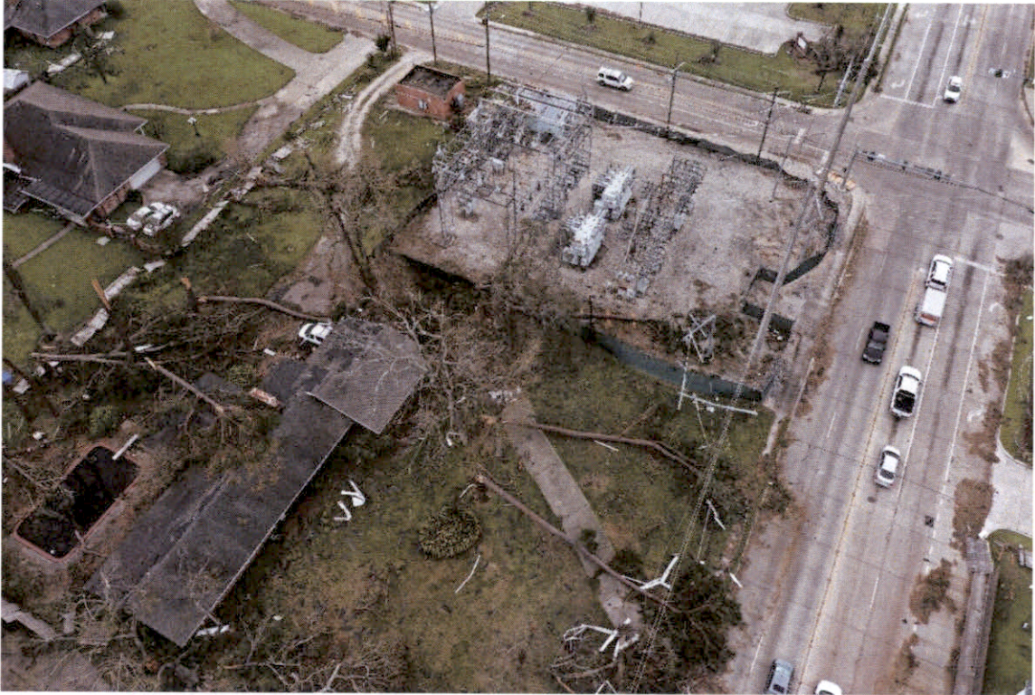
Figure 4-11. Trees Damaged near Transmission Line
