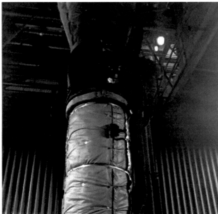
Figure 11: Heated Blankets on Cones Downspout of Silos
